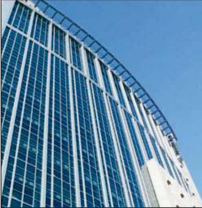
Top portion of photo shows a curved screen canopy at the 16 th floor level equipped with a Pro-Bel aluminum monorail system which is used to suspend a 30'-0" (9.1 m) 'F' Type platform (4 point suspension). U.S. Courthouse & Federal Building, Sacramento, California.
