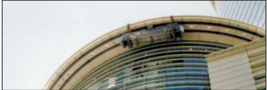
Platform is suspended from trolleys secured to soffit mounted steel I-beam monorail. Recessed facade at upper level requires platform to be switched from an interior monorail to an exterior monorail and vice versa using a turning hub or “turntable” (see close-up photo below, right). Enron Building 2, Houston, Texas.
