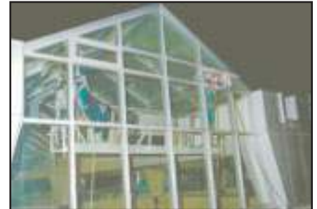
Localized operable window is used to access monorail for securing platform suspension lines.
