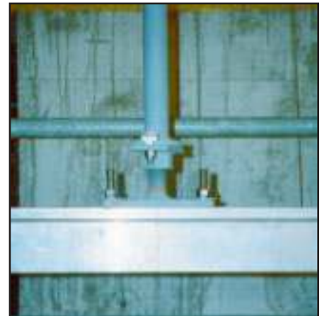
Adjustable monorail hanger, secured to structure above, allows for accurate leveling of rail.
