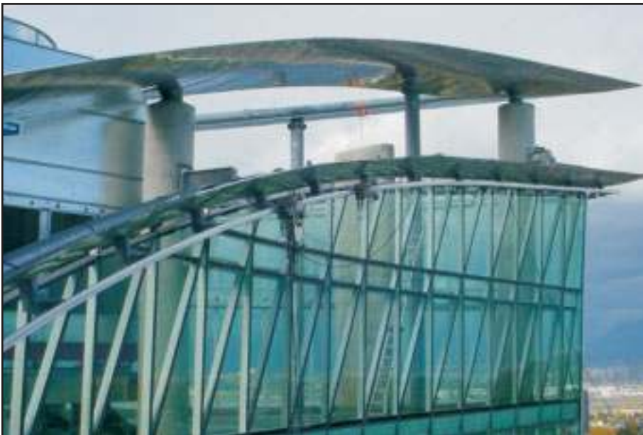
The top of this curved building elevation shows a monorail utilizing electric powered trolleys to pull a platform (not shown) up the incline. See close-up photo of motorized trolley in center of page. Surrey City Centre, Surrey, British Columbia.
