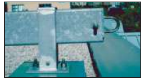
Outboard end of beam equipped with stainless steel U-bar. Bolt at inboard end and stop plate at inboard end prevents beam from sliding out of yokes.
