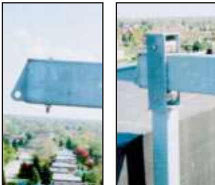
Beam end (left) shows suspension shackle plate and bolt-type stop. Steel pier (right) shows stainless steel rollers that provide for easy beam movement.
