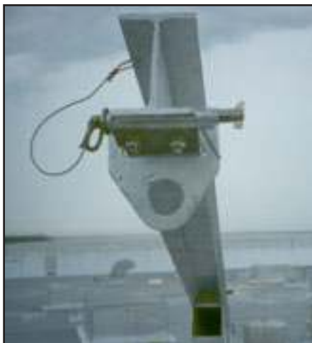
Photo (left) shows outboard end of outrigger equipped with trolley for attachment of primary suspension line. Stainless steel locking pin tethered to beam locks trolley in desired position.
