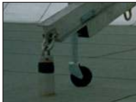
Outrigger tie-back anchor (Pro-Bel EPB Series roof anchor). Separate independent lifeline anchor is same type.
