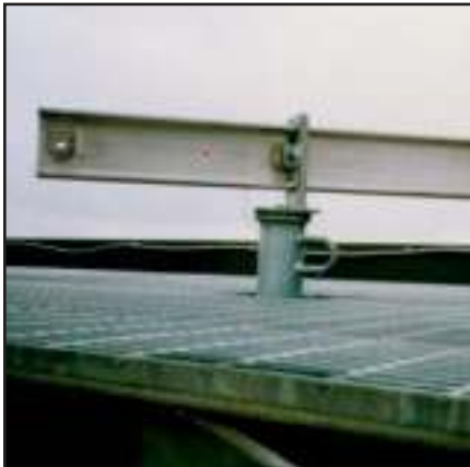
Inboard end of outrigger beam is equipped with a swivel-type adapter and safety anchor attached to the beam base.
