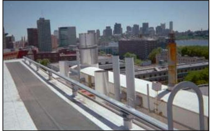
View of penthouse roof in photo at left shows rail support piers located at 10'-0" to 12'-0" (3050 mm to 3658 mm) centers. Black walkway strip on roof protects single ply roof membrane from roof traffic i.e. window cleaners or other maintenance personnel.
