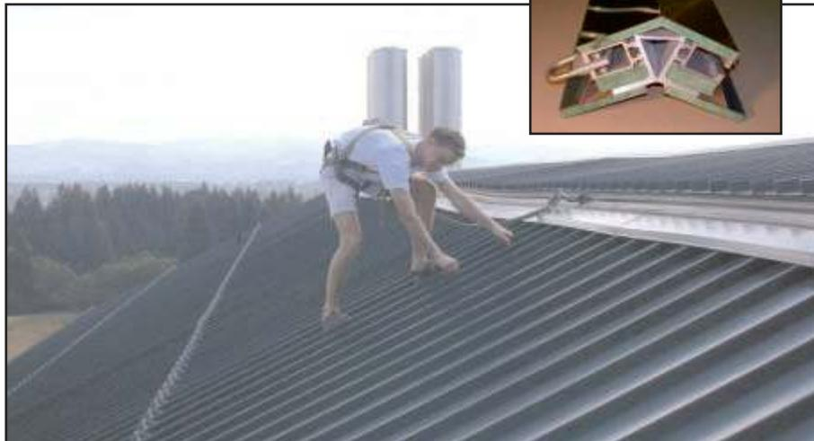
Photo shows a Pro-Bel ridge mounted type of trolley rail designed for the maintenance of a peaked roof. Worker's safety lifeline is secured to a stainless steel U-bar trolley located either side of the rail. The worker or several workers are able to traverse horizontally to any point on the roof, W.S.U. Physical Plant, Washington State University. Inset is product design photo of trolley rail.
