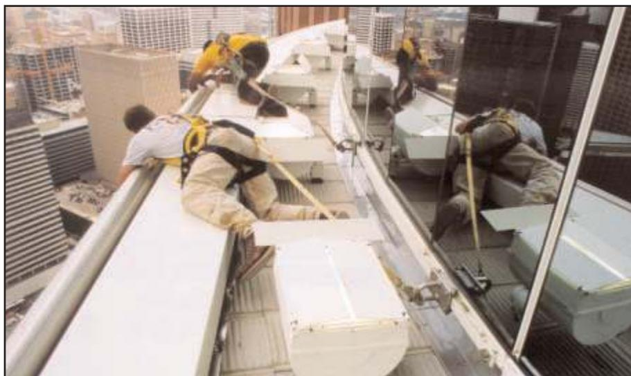
Rail mounted Pro-Bel trolley system at base of windows in this 40<sup>th</sup> floor Tower application is used to secure workers' fall protection lanyards enabling service to any part of narrow roof areas. Enron Building 2, Houston Texas.
