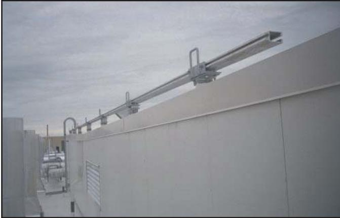
This unusual penthouse roof mounted rail is equipped with yokes for securing the inboard ends of long reach outrigger beams. The working ends of the outriggers are supported on a high parapet wall (not shown). Rolling trolleys inside the rail are used for workers' lifelines.
