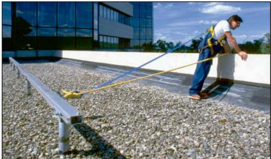
Roof mounted horizontal aluminum rail. Photo shows worker preparing to work over parapet. Both lines are secured to rolling trolleys. Parapet to support 1800 lbs (7.9 kN) vertical load.
