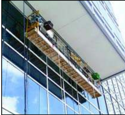
This exterior Pro-Bel aluminum concealed soffit monorail provides ease of access to the overhang area above for the glazing contractor. Soffits/ceiling must be hung independently to avoid potential for damage from deflection when rail is under load. Air Canada Centre, Toronto, Canada.
