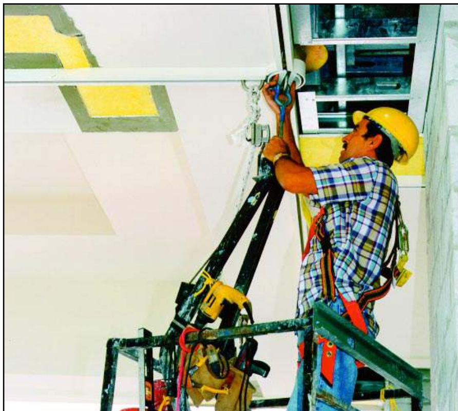
This photo shows worker finishing ceiling around Pro-Bel monorail and corner-turning hub while working from a single work cage. The hub facilitates automatic turning at corners. Diplomat Hotel Resort, Hollywood, Florida.
