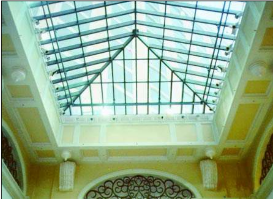
Atrium showing perimeter standard monorail blending in with aluminum clad steel rafters. Separate monorail is located at ridge point. For window cleaning, platform can be suspended at any desired angle or height around all four sides of atrium glass. Beau Rivage Hotel, Biloxi, Mississippi.
