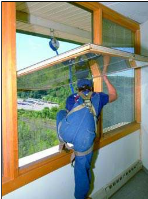
Access to exterior monorail is achieved via a localized operable window. This worker has a wide spandrel ledge to step onto, however a separate and independent fall arrest system secured to an interior safety anchor is normally required to safely connect to the monorail (continuous protection).
