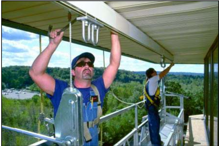
Workers adjusting new Pro-Bel exterior monorail system which accommodates four trolleys for a two person platform (two for suspension of the platform and two for worker's lifelines). Suspension cable is temporarily secured to the structure above the soffit to facilitate installation. Monorail has been powder coated to match soffit finish. Overlook at Great Notch, Little Falls, N.J.
