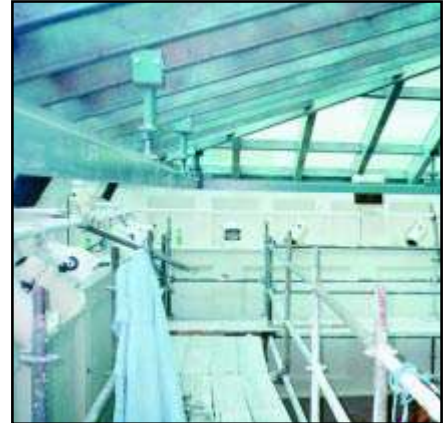
Construction photo shows adjustable monorail hangers secured to steel rafters.
