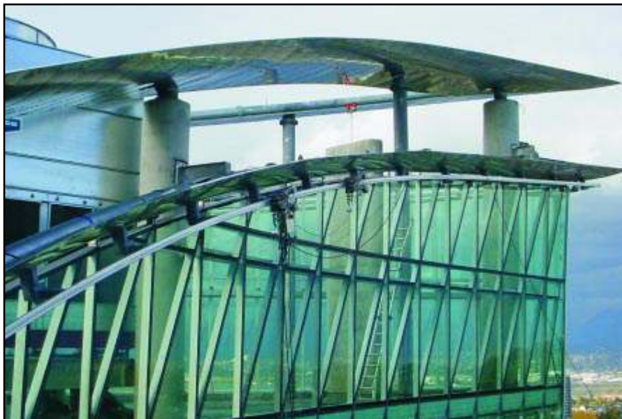
The top of this curved building elevation shows a monorail utilizing electric powered trolleys to pull a platform (not shown) up the incline. See close-up photo of motorized trolley in center of page. Surrey City Centre, Surrey, British Columbia.
