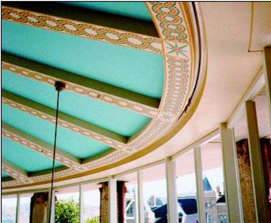
Pro-Bel monorails are often installed in decorative ceilings. This curved monorail forms a complete circle. Salt Lake City Courthouse, Utah.
