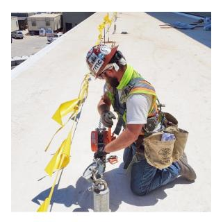
Bel, partially certified or uncertified anchors can be used by implementing a combination of: performance engineering, alternative work practice techniques and administrative controls; in order to provide sufficient protection to workers and ensure proper use with the limitations identified in a work plan.
