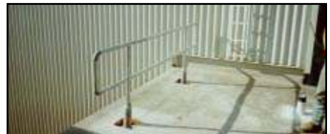
Localized railings provide added protection near access hatches, doors, and/or around mechanical equipment.
