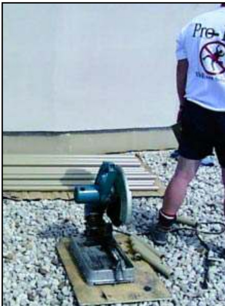
Pro-Bel installers cut the horizontal rail on site to length as required.
