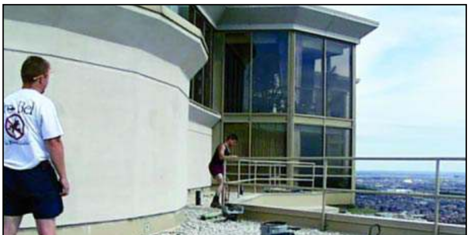
Pro-Bel installers adjust corners and horizontal top rail to ensure guardrail is level and square before tightening up vertical posts.
