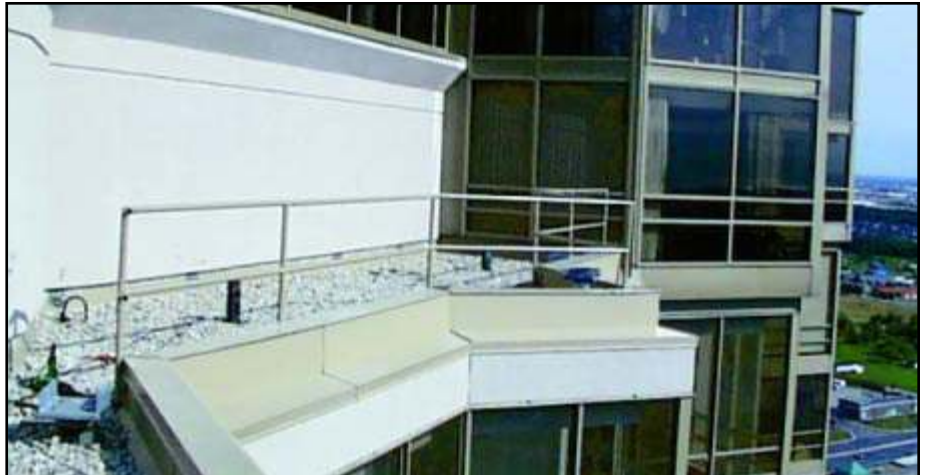
The angular roof line required complete perimeter protection. This Photo shows partial installation of Pro-Bel safety railing to inside of parapet wall.
