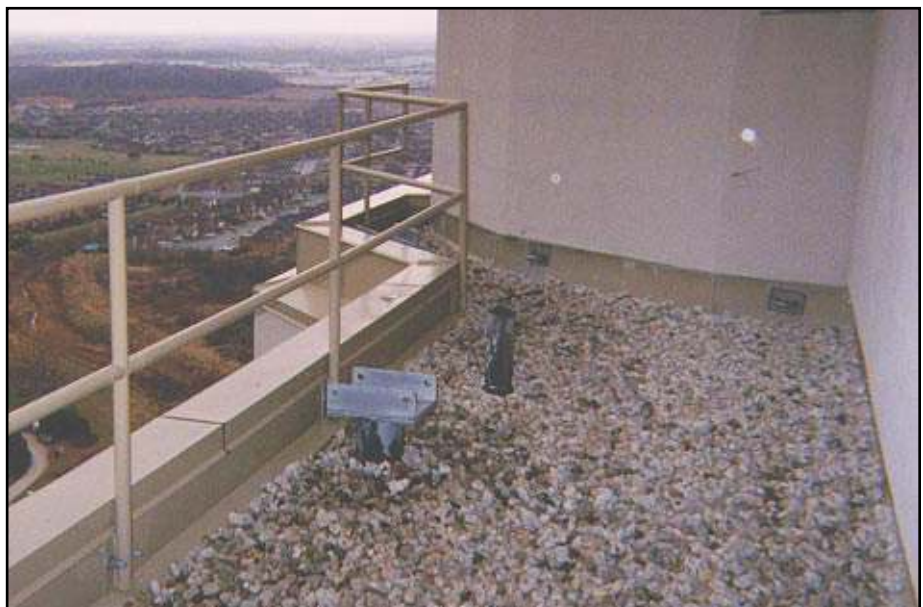
Safety guardrail at davit base anchorage which is used for suspended maintenance. Low parapet requires 42" (1067 mm) high guardrail if workers are approaching within 6'-0" (1830 mm) of roof edge. This installation is located in a narrow roof area.
