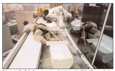
Rail mounted Pro-Bel trolley system at base of windows in this  $40^{\rm th}$  floor Tower application is used to secure workers' fall protection lanyards enabling service to any part of narrow roof areas. Enron Building 2, Houston Texas.
