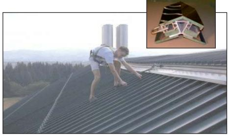
Photo shows a Pro-Bel ridge mounted type of trolley rail designed for the maintenance of a peaked roof. Worker's safety lifeline is secured to a stainless steel U-bar trolley located either side of the rail. The worker or several workers are able to traverse horizontally to any point on the roof, W.S.U. Physical Plant, Washington State University. Inset is product design photo of trolley rail.
