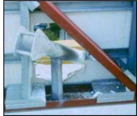
The two construction photos above show a curved horizontal rigging sleeve anchored behind a screen wall on the roof and passing through both the wall and a soffit roof. At rear of sleeve a primary line and lifeline are typically shackled to the two straight bars.
