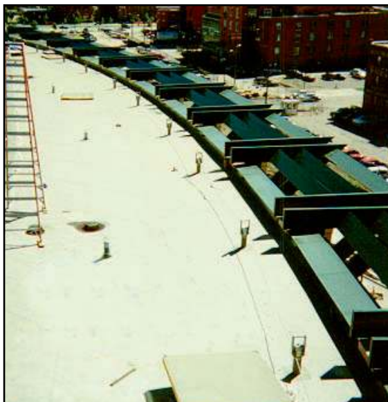
Construction photo showing Pro-Bel roof type rigging sleeves. Pepsi Center, Denver, Colorado.
