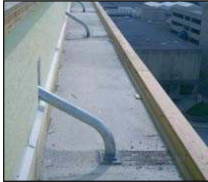
The two construction photos above show a curved horizontal rigging sleeve anchored behind a screen wall on the roof and passing through both the wall and a soffit roof. At rear of sleeve a primary line and lifeline are typically shackled to the two straight bars.
