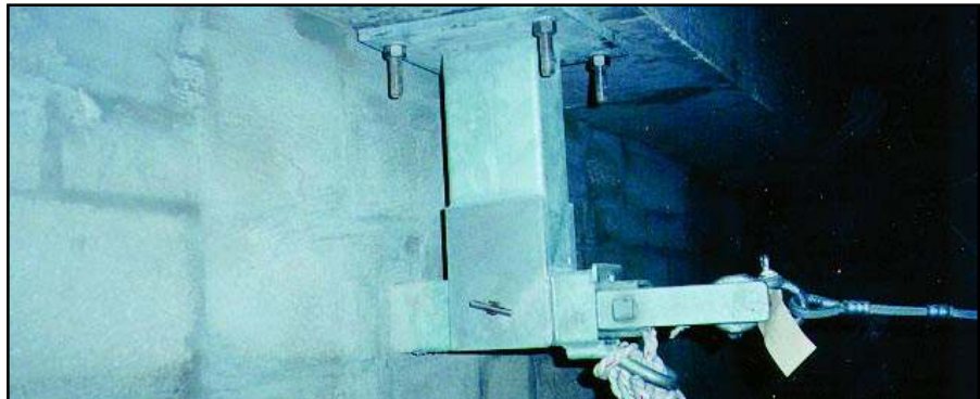
Horizontal rigging sleeve (in service position) is anchored to concrete roof beam and tied back to an interior wall mount safety anchor using steel cable. Worker's rope lifeline, tied to U-bar safety anchor, passes through sleeve to exterior.
