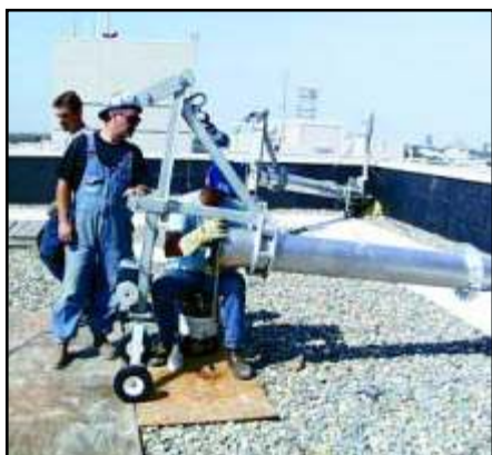
Annual maintenance and inspection is required in order to comply with OSHA and ANSI/IWCA I-14.1 requirements.
