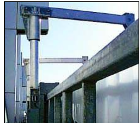
Square tubular wall mounted track supporting a motorized davit system. Islip Courthouse, Islip, New York.
