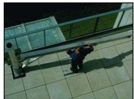
4. Aluminum boom is mechanically fitted to mast and secured with stainless steel connecting pins.
