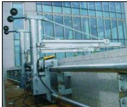
Parapet wall mounted motorized davit system, George's Quay Development, Dublin, Ireland.
