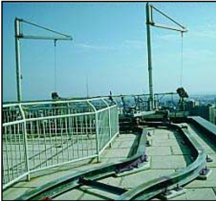
Motorized rolling davit system utilizing I-beam tracks.
