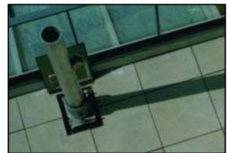
3. Aluminum mast is set into socket and twist locked into place.
