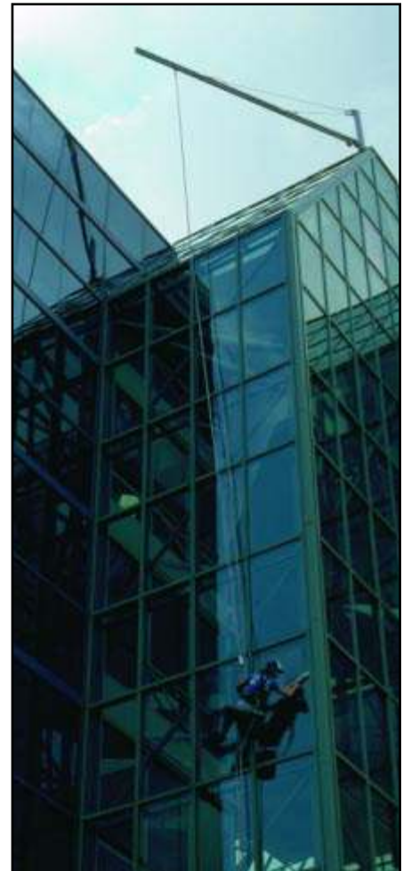
Working down face of building using Pro-Bel long span davit boom and bosun's chair. Bull Corporate Centre, Toronto, Ontario.
