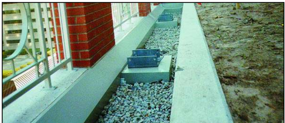
Concrete pier mounted davit bases shown in this photo are concealed in planter boxes.
