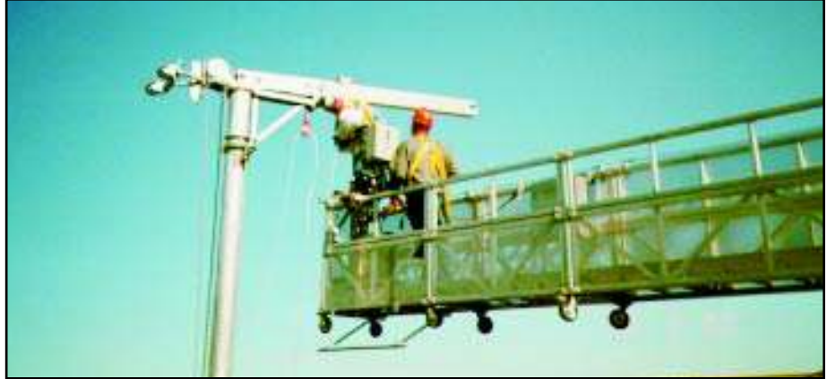
This photo shows Pro-Bel installers maintaining the manual chain driven trolley during the roof rigging process. U.C. Davis Medical Center, Sacramento, California.
