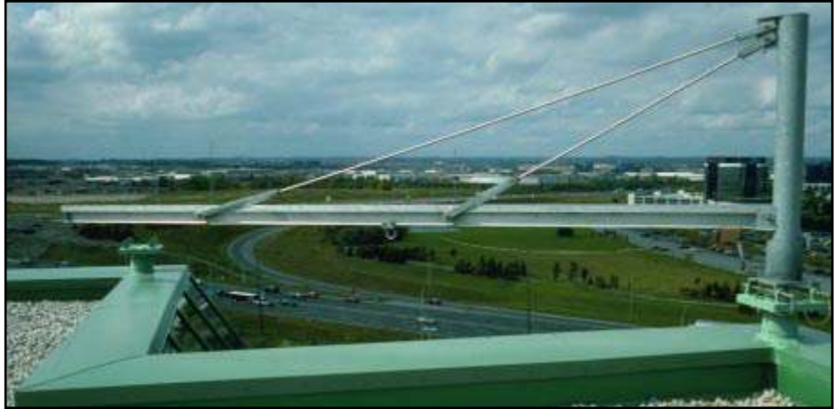
Portable 21'-0" (6.4 m) long reach davit arm is employed for sloped glass and designed to suit bosun's chair equipped with descent control equipment.
