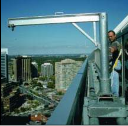
Rolling davits are designed for roofs with restricted access or long reach rigging options. Worker is shown manually positioning davit. Motorized models are also available. Worker's lanyard is clipped to U-bar safety anchor welded to rolling carriage. 25 Sheppard Ave., Toronto, Ontario.
