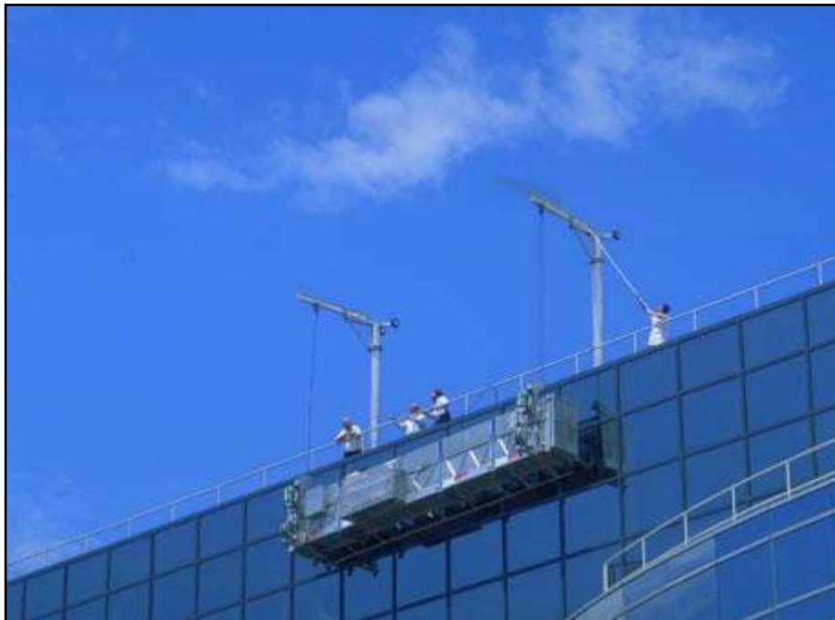
This Pro-Bel roof rigged davit system suspends a permanent powered platform system. Bose Corporation, Boston, MA.
