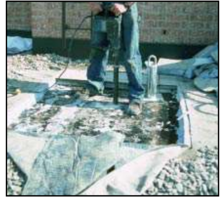
2. Holes are drilled into or through concrete deck to accommodate roof anchor bolts.
