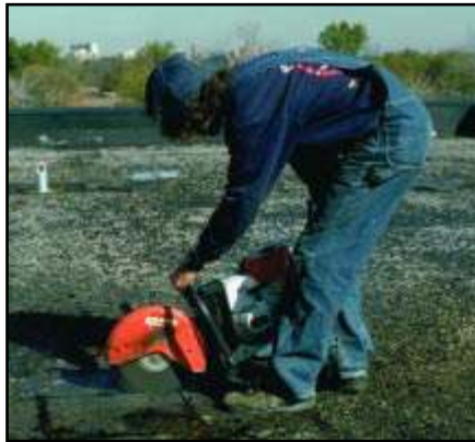
1. Small area of roof covering is removed down to concrete deck.
