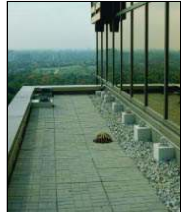
This narrow roof area requires anchors on 5'-0" (1830 mm) centers. See Anchor Spacing Chart below.
