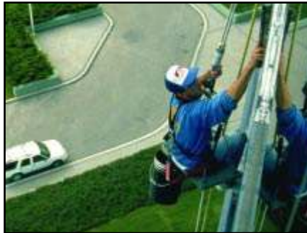
Bosun's chair is the equipment of choice among window cleaners. Pro-Bel safety anchors (see photo at right) are used to secure chair and separate lifeline.
