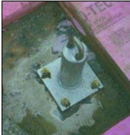
3. Anchor is installed using either bolt-through or chemical adhesive securement depending on access from below.
