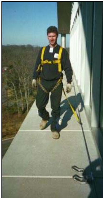
Worker above uses Pro-Bel "Hands-Free" horizontal lifeline cable to safely access recessed windows as well as custom ledge-mounted Pro-Bel safety anchors (one for bosun's chair and one for lifeline) for "drops" below.
