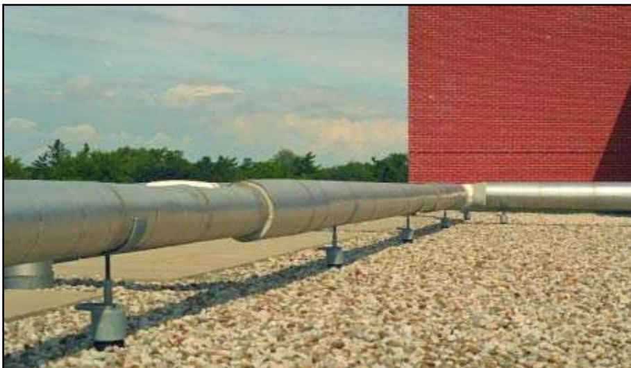
Pro-Bel galvanized steel pipe support complete with U-Bar safety anchor.
