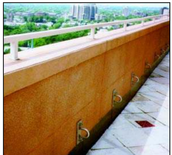
Series of Pro-Bel wall anchors bolted to structural concrete parapet, used to secure a bosun's chair suspension line and workers' lifeline (interchangeable).
