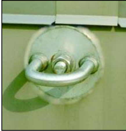
Pro-Bel PB type wall anchor in concrete wall of rooftop mechanical room.
