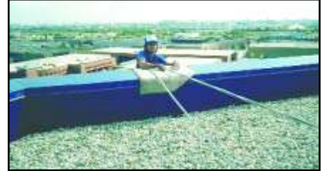
The chair is rigged directly to an anchor in line with the point of suspension. A separate independent anchor on the roof is required to secure the worker's fall arrest lifeline.
