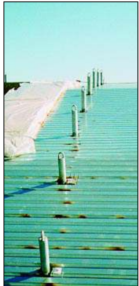
This photo shows a Pro-Bel roof anchor installation. Anchors are welded to structural steel before a horizontal lifeline cable system is installed to provide fall protection on this arched roof.
