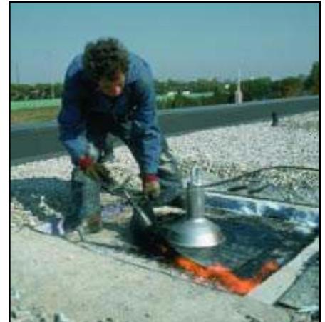
4. Watertight integrity of roof is restored using spun aluminum flashing and new roof covering (roof patch). Photo shows protected membrane roof.
