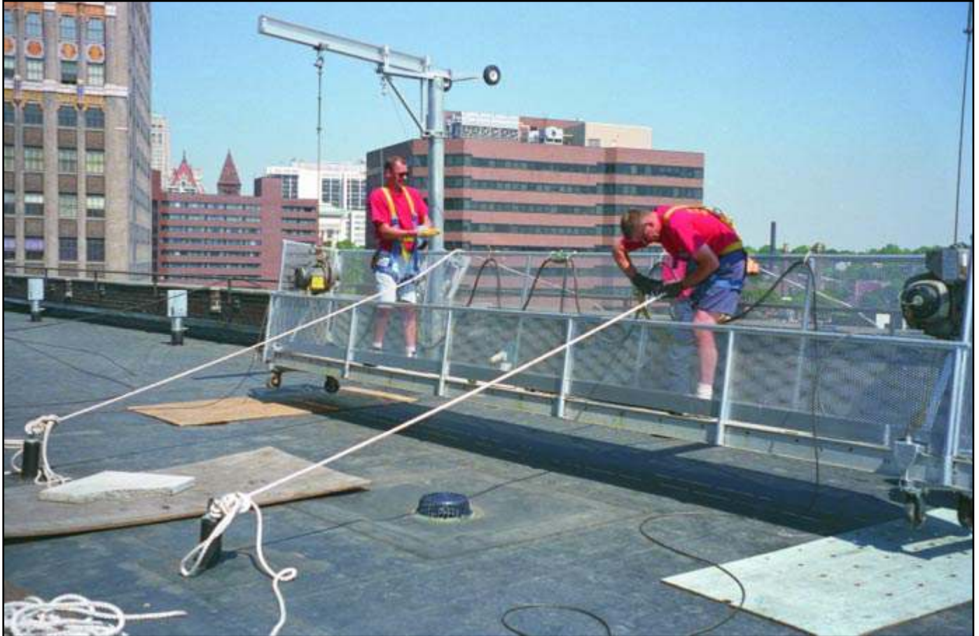
Window cleaners preparing to launch a contractor supplied platform over a parapet wall using Pro-Bel davits with rotating heads. Steel cables are used to suspend the platform while workers are tethered to independent Pro-Bel roof anchors with rope lifelines.
