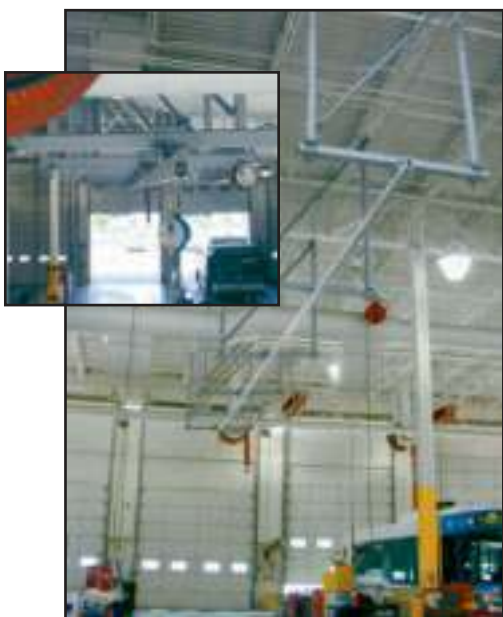
Pro-Bel overhead trolley rail (with retractable lanyard, inset) is used for fall protection while servicing top of vehicles in bus bay garage.
