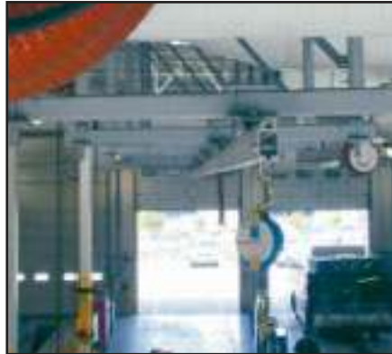
Retractable lanyard secured to Pro-Bel overhead trolley rail (bus garage).
