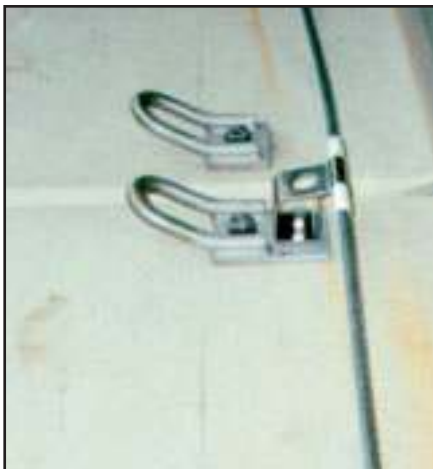
Typical Pro-Bel ledge anchor which is accessed via a horizontal cable lifeline ("Hands-Free" system at intermediate bracket shown).
