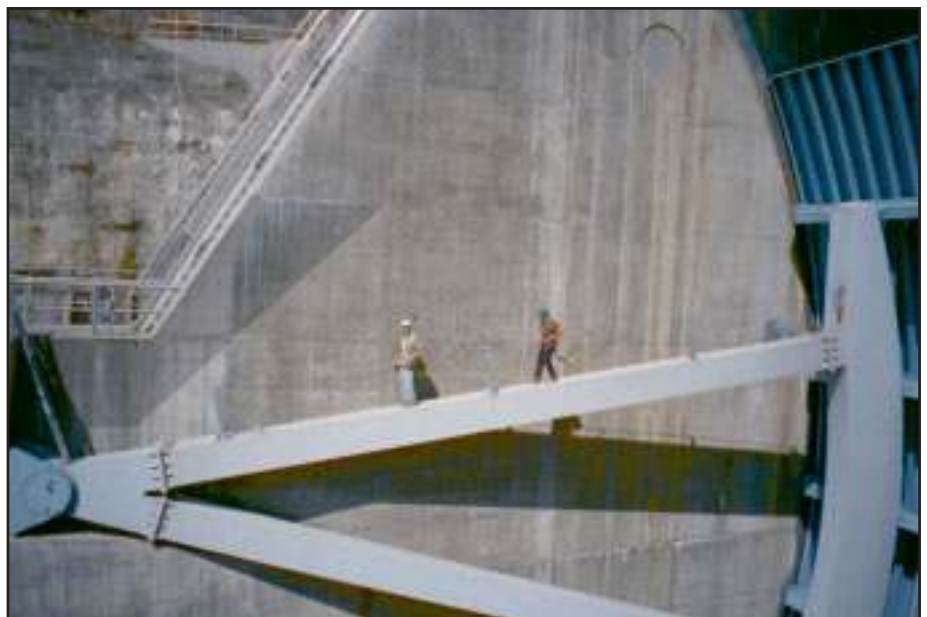
Spillway fall protection system at GMS/Bennet facility shown in photo on page I-2. Pro-Bel Horizontal Cable System is employed to safely traverse the spillway arm which is 70'-0" to 90'-0" (21.3 m to 27.5 m) above the spillway concrete surface below.
