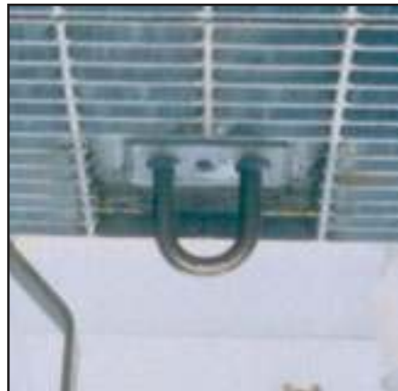
Typical Pro-Bel catwalk anchor. Can be secured to all types of metal surfaces.
