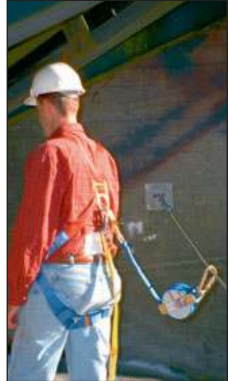
Retractable lanyard secured to body harness with other end secured to single span Pro-Bel horizontal cable lifeline system. GMS/Bennet Dam.
