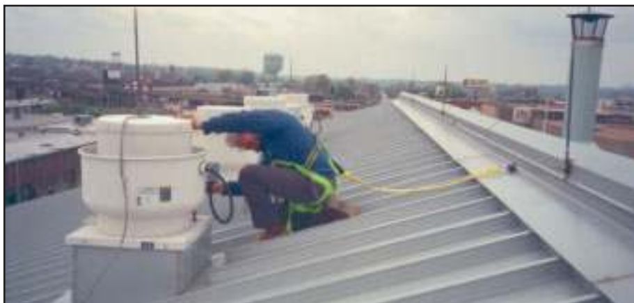
Pro-Bel "Hands-Free" Horizontal cable lifeline provides 100% continuous protection for electrical, mechanical and roof inspection maintenance, and access to window cleaning, exterior maintenance, tie-back, and lifeline anchors when necessary.
