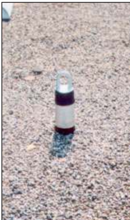
Pro-Bel PBE Series roof anchor with heat-shrink rubber collar flashing.
