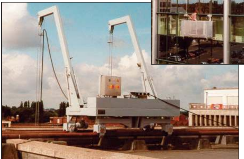
A variation of Pro-Bel Model FS-3000 Trolley Roof Car. Trolleys are supported on 4 wheel assemblies operating on galvanized pipe rails mounted on concrete piers cast into the roof slab. Steel base and suspension jibs have 360° slewing and luffing capability.
