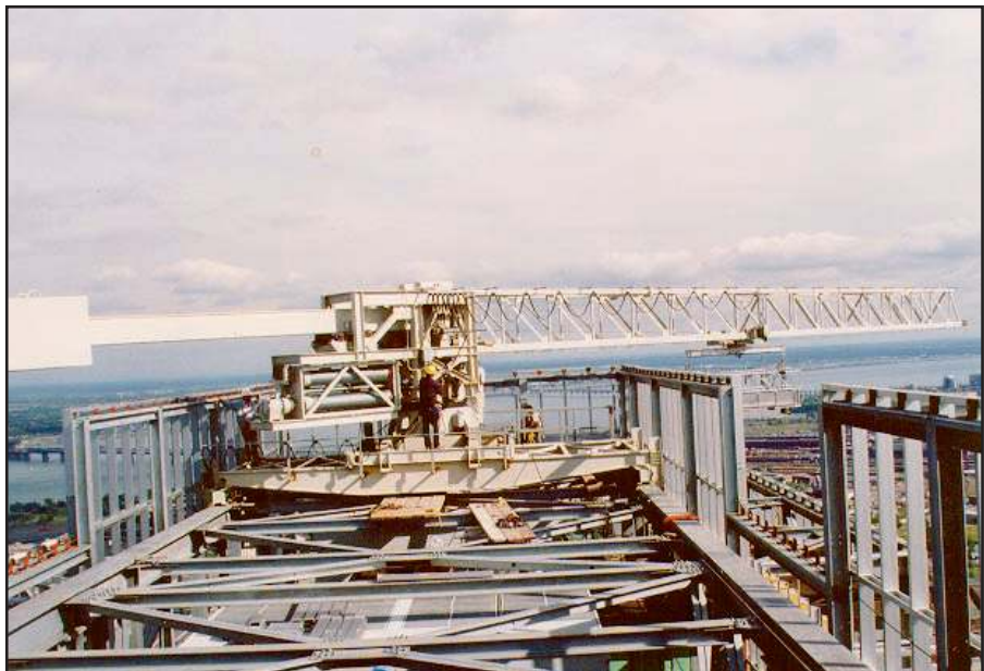
This roof car, located on the roof of a 47 storey tower with a very complex building geometry is equipped with an 84'-0" (25.6 m) long slewing boom and travels in two directions on I-Beam rails. A pivoting trolley that moves along the full length of the boom is used to suspend the platform. 1000 De La Gauchetiure, Montreal, Quebec.
