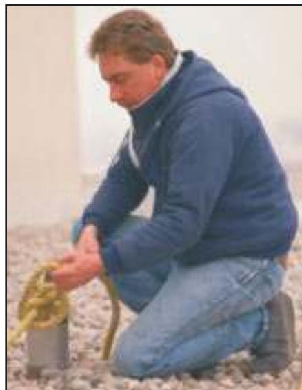
Pro-Bel safety anchors may be used for securing lifelines, as a tie-back for primary rigging equipment or to directly rig (secure) a bosun's chair. Anchors protect workers' lives in case the suspension equipment fails, or in the event a worker momentarily loses control.
