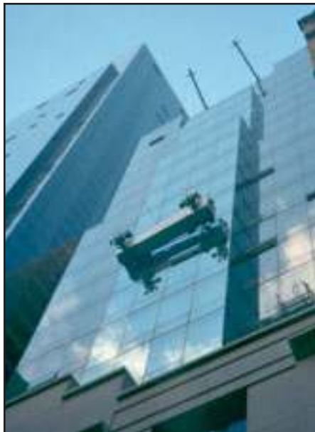
This Pro-Bel permanent powered platform employs Pro-Bel 14'-0" (4.3 m) long span davit booms to clear roof terraces and cornice at lower level. The Millennium building, New York, NY.
