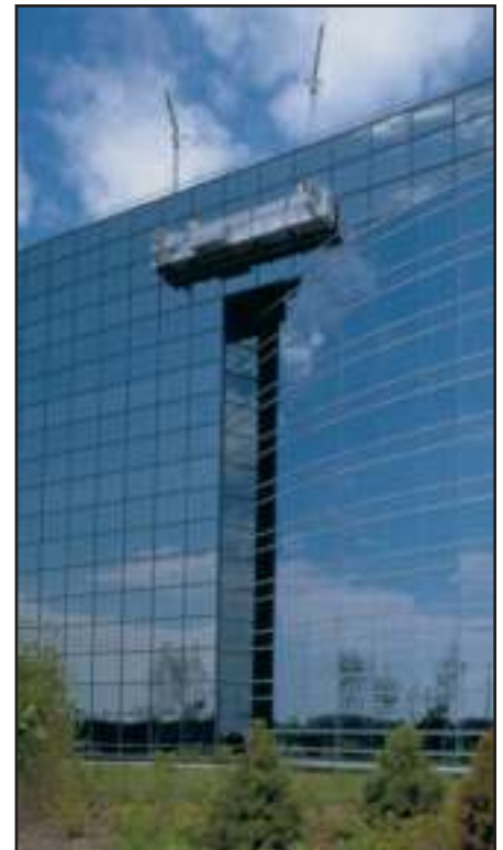
Pro-Bel modular powered platform system suspended via a roof rigged davit assembly.
