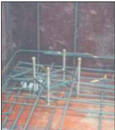
Pro-Bel davit cage cast into concrete slab by General Contractor.
