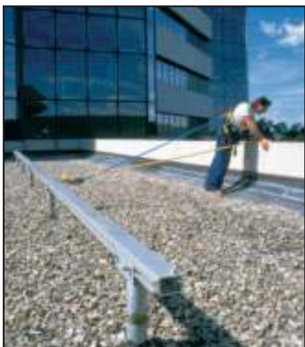
Monorail can also be roof mounted (as shown) or wall mounted to suit application.
