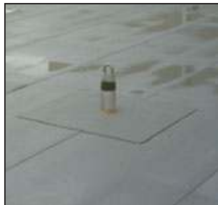
Single ply roof showing typical Pro-Bel roof anchor. Reliable flashing/sealing techniques are employed to satisfy virtually any roof membrane condition.
