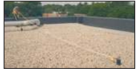
Anchors are also used to secure workers approaching the roof edge when parapet wall is less than 42" (1067 mm) guardrail height.
