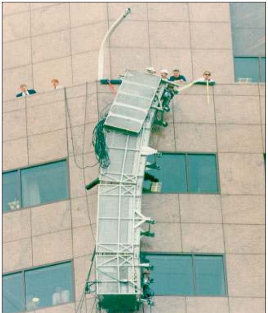
In this window washing accident, one end of the platform broke loose and one window cleaner fell to his death while a second man was saved by his independently anchored rope lifeline.
