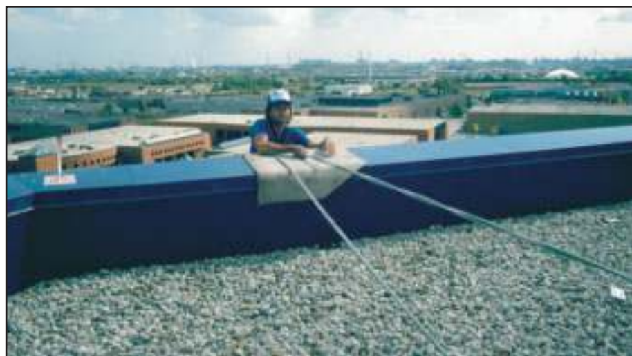
Parapet wall must be strong enough to support applied loads of suspension ropes, wall clamps/hooks or outrigger beams with counterweights. Alternatively, a portable davit arm or outrigger beam dolly can be used to clear the parapet.
