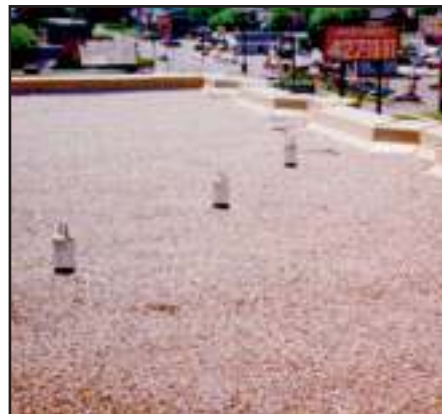
Due to stringent government standards, anchor placement requirements i.e. in line with the point of suspension and free fall distance, anchors must often be placed on the roof.
