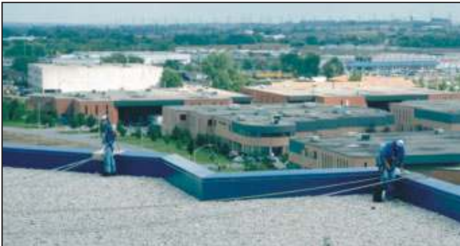
Two window cleaners are shown direct rigging to separate and independent roof anchors.
