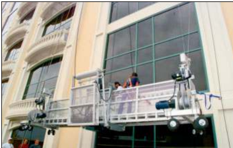
Extreme right and left hand side of photo shows how platform is stabilized against wind using cable, down rigged lines anchored to a Pro-Bel anchor at ground level and davit arm at roof level. Nylon webbing stabilizer ties secure the platform to down rigged lines—a custom, restrictive solution designed with a slip rope grab to control amplified loads.
