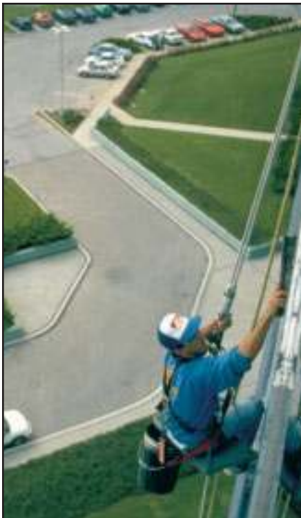
Pro-Bel safety anchors, in addition to securing worker's lifelines, are a practical means of suspending a bosun's chair equipped with a descent control device.
