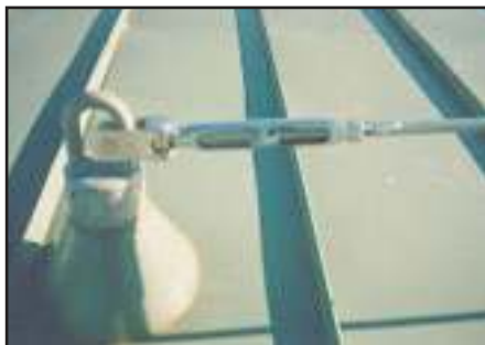
Standing seam sloped metal roof showing end tensioner and roof anchor terminal of Pro-Bel Horizontal Cable Lifeline System.
