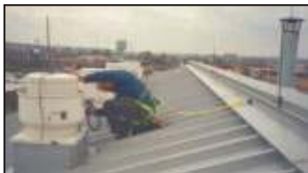
Metal roof maintenance and electrical/mechanical roof inspection performed safely while tied to horizontal lifeline cable.
