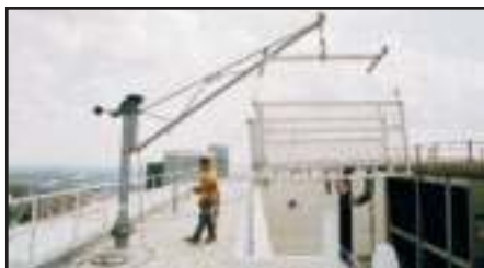
The platforms are suspended from trolleys mounted inside monorails located on soffit overhangs at the uppermost level of the buildings. Recessed balconies or building faces at the upper levels require platforms to be switched from an interior monorail to an exterior monorail and vice versa using a "turntable." To avoid using a perimeter-type electrical bus bar system of providing power to the platforms, battery powered trolleys are used at each platform "drop". The batteries are plugged into permanent electrical outlets located in soffits when not in use.
