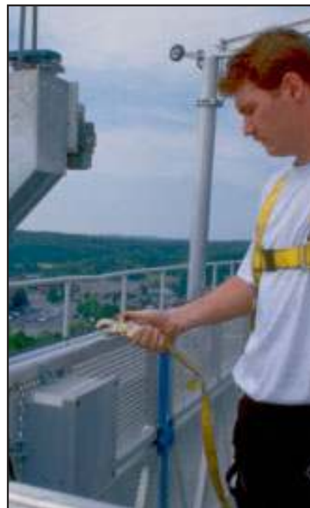
Four point suspension platforms include a permanently installed horizontal cable system (dog line) for the attachment of workers' fall arrest lanyards (no separate hanging lifelines).
