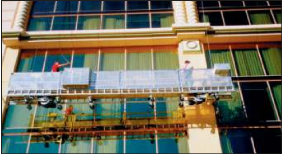
This Pro-Bel modular aluminum platform is suspended from a Pro-Bel motorized traversing davit system which moves on a custom, narrow, double I-beam track at roof level. Sun-Coast Casino and Hotel, Las Vegas, Nevada.
