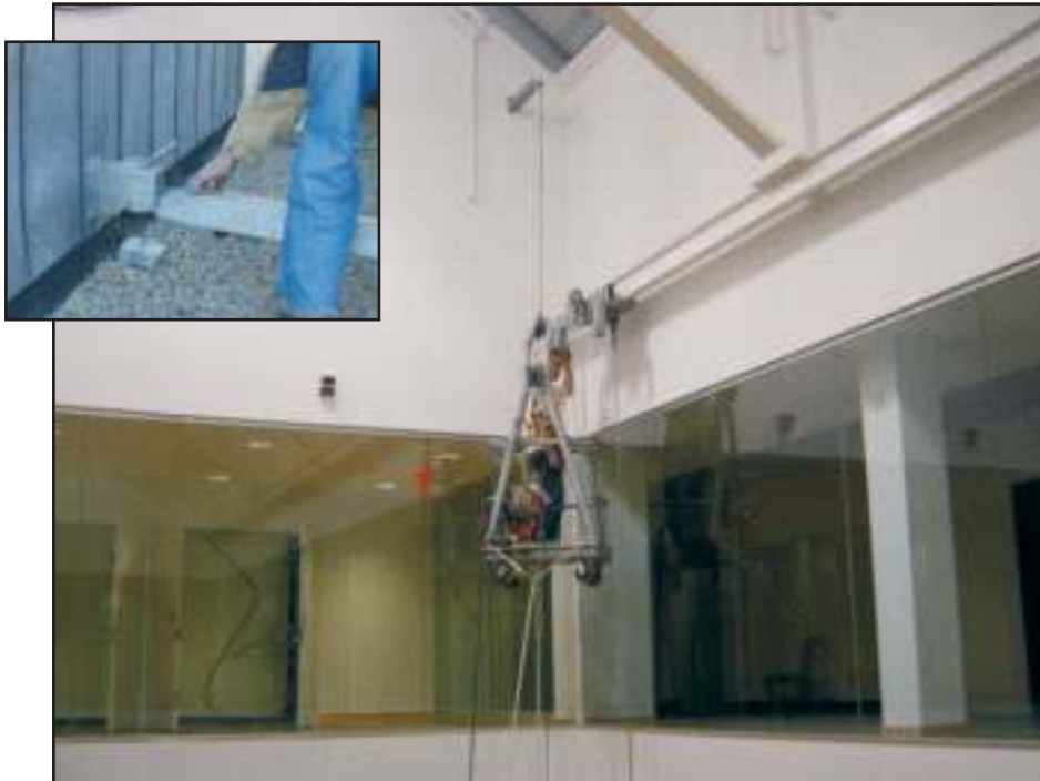
In the photo above, the suspension cables for the telescoping platform are attached to the rolling trolley equipment by first lowering a suspension line through the rigging sleeve penetrating the top of the atrium. The line is used to raise a single work cage carrying the suspension cables to the trolleys. Inset photo shows rigging sleeve being inserted through the atrium wall from an adjacent roof.
