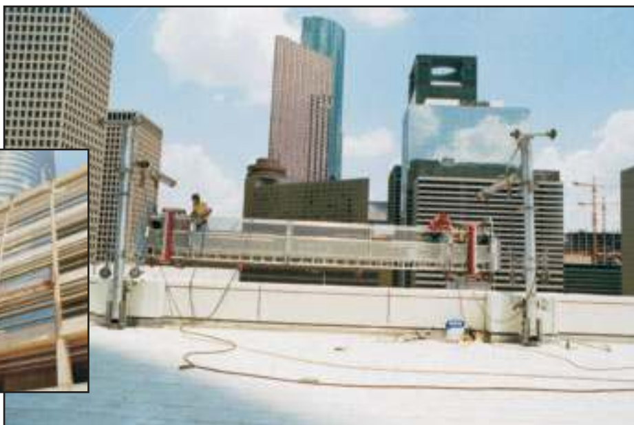
Pro-Bel davits 14'-5" (4.4 m) high with 11'-7" (3.5 m) reach located on 8 th Floor Podium are used to suspend one of a variety of different sized platforms. Inset shows platform traveling down face of Podium.
