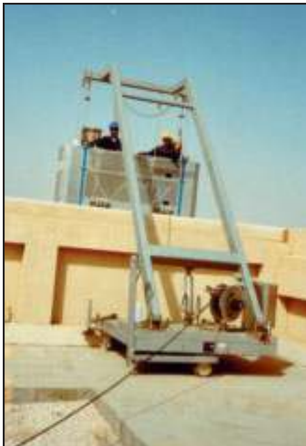
Pro-Bel Model PT 3008 Roof Car (Powered Trackless Trolley) is supported on hard rubber tired wheels and operates on a reinforced concrete bearing surface (or similar) cast on top of the roof finish. Steel base frame and suspension jib have 360° slewing and luffing (up and down) capability.
