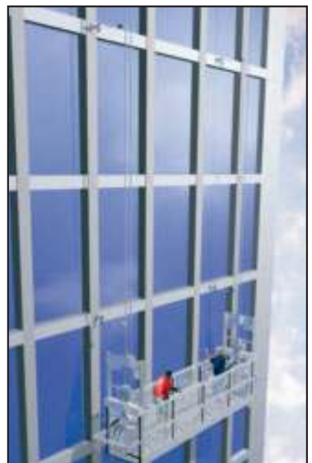
As a platform descends past the elevation of a tie-in guide, each of the platform's two occupants secure a stabilizer tie between a platform suspension cable and a detent pin or button.
