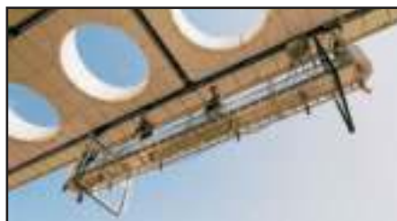
On the Enron Tower, the 3 sequence photos show an unusual procedure requiring a Pro-Bel winch-hoist and special lifting frame be used to hoist platform sections from a Tower roof storage area, swung across a narrow terrace, and then lowered through a 10'-0" (3 m) diameter opening in the unique roof overhang, to the 40 th floor balcony landing areas where the platform sections are assembled and launched. The bottom photo shows the assembled platform suspended from a monorail and battery operated trolley system.
