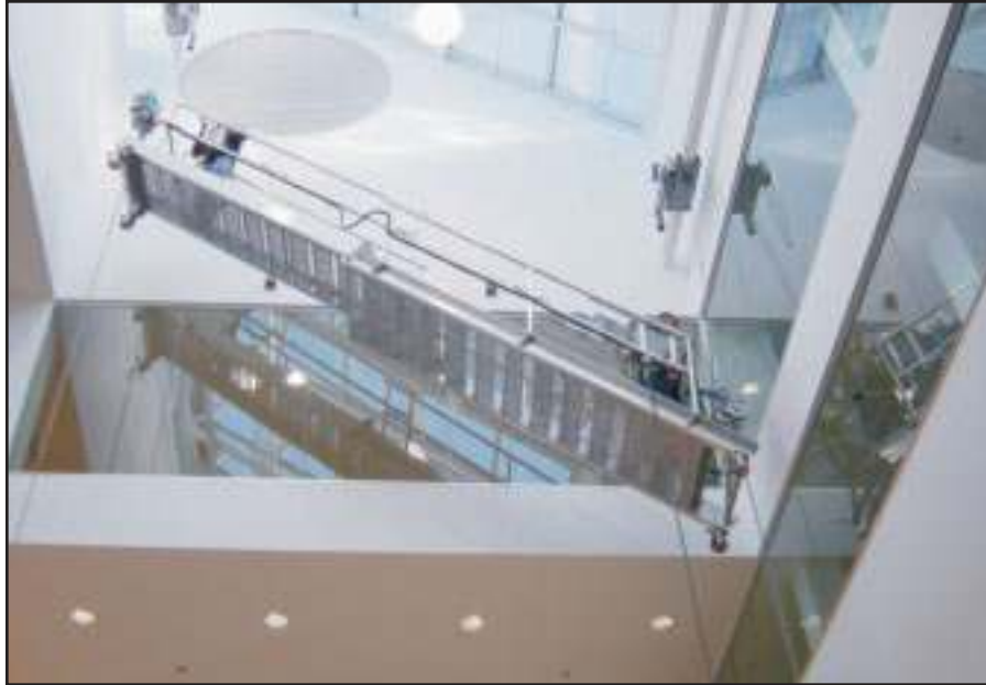
This unique project employs a Pro-Bel motorized telescoping platform to access the sloped interior atrium glass. Suspended from trolleys mounted on I-beam supports, the platform can traverse horizontally as well as up and down while the telescopic feature permits the platform to be narrowed or lengthened as required in order to service the variable atrium spaces. Hartford Public Library, Hartford, Connecticut.
