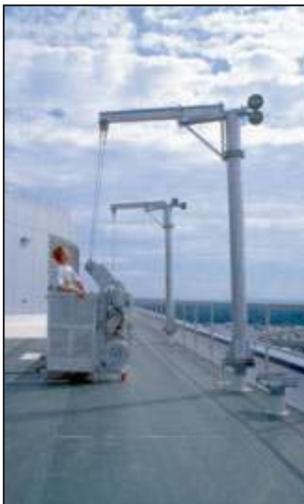
Rooftop photo shows rotating davit arms turned inwards. Platform is raised via two hoist motors mounted on the low profile walk-through stirrups, then pushed outwards to clear the parapet/safety rail.
