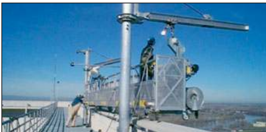
Using the rotating davit arms, the platform is swung across the catwalk and over the parapet, and then rolled out on the booms using stainless steel trolleys. Note the custom fitted face roller extensions mounted on the platform rail.
