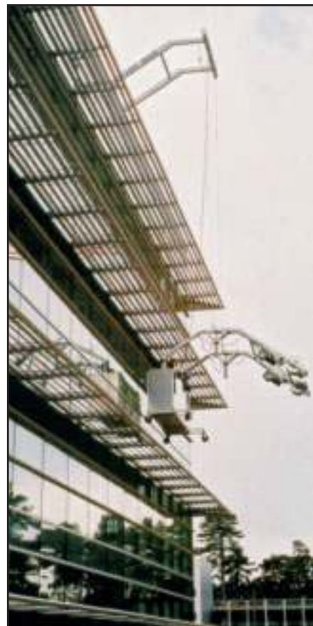
This platform utilizes a counterbalance or counterweight concept to help move the platform inboard of the suspension points which is very useful for reaching the glass under the sunscreens in this application. The platform moves laterally via a roof car thereby allowing convenient sideways movement controlled from the platform.
