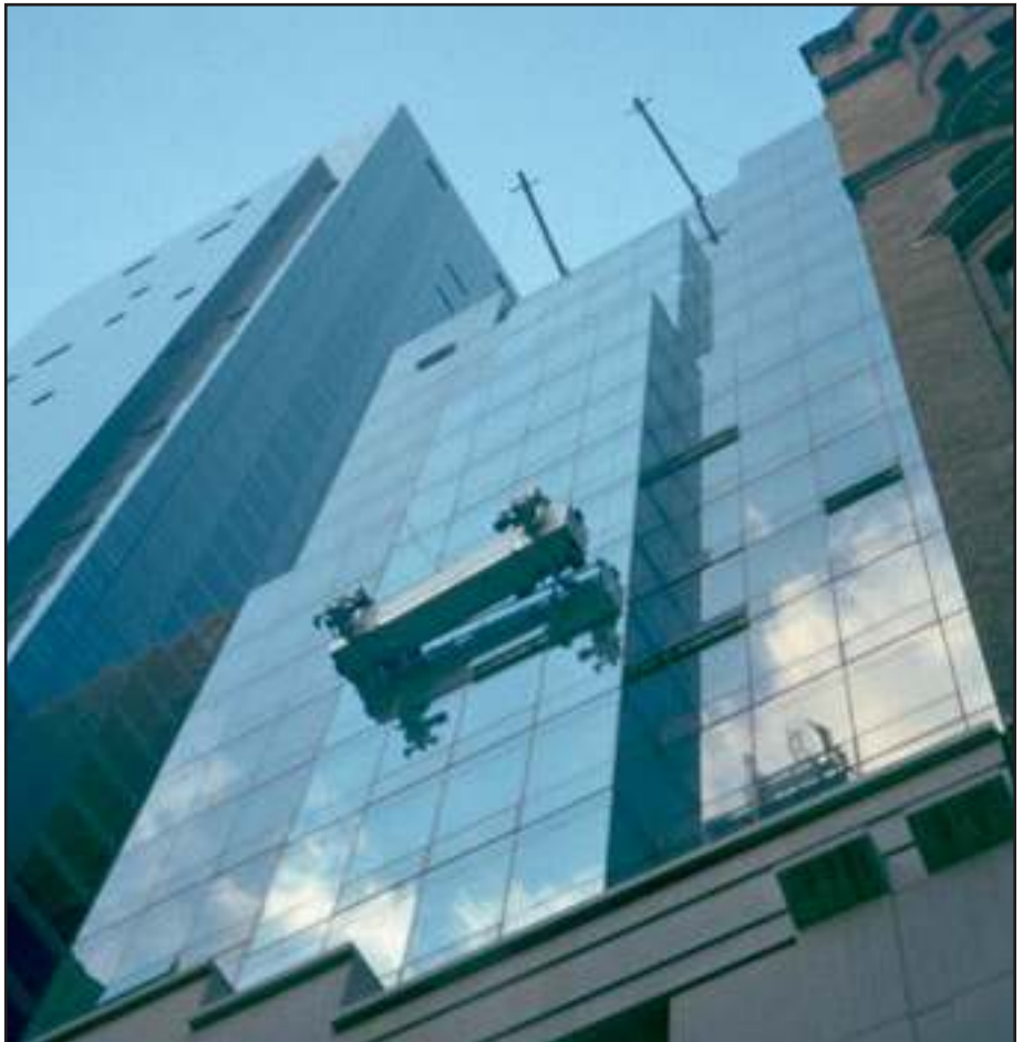
This Pro-Bel powered platform employs Pro-Bel 14'-0" (4.3 m) long span davit booms to clear roof terraces and cornice at lower level. The Millennium building, New York, NY.
