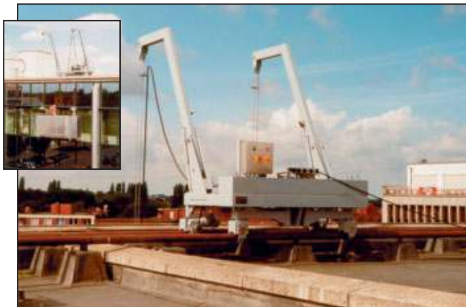
A variation of Roof Anchored Trolley Roof Car. Trolleys are supported on 4 wheel assemblies operating on galvanized pipe rails mounted on concrete piers cast into the roof slab. Steel base and suspension jibs have 360° slewing and luffing capability.
