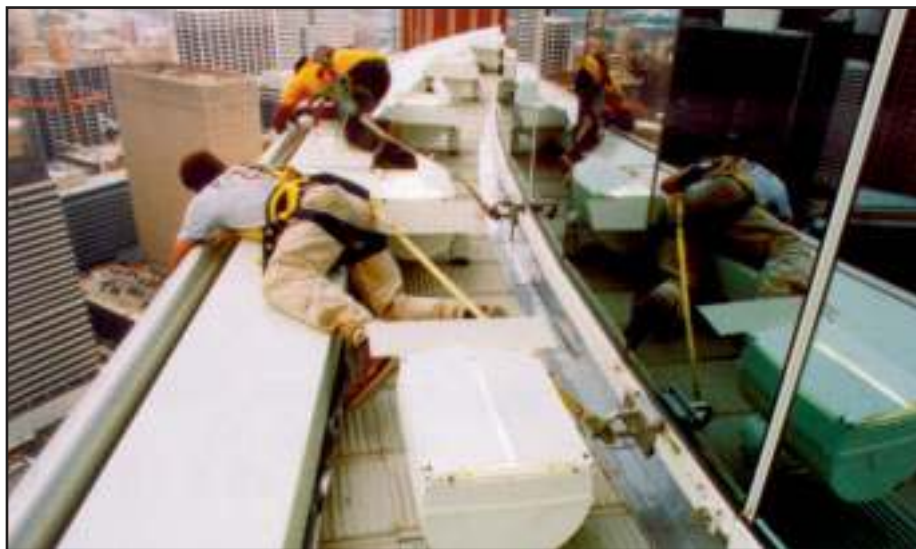
Rail mounted Pro-Bel trolley system at base of windows in this 40 th floor Tower application is used to secure workers' fall protection lanyards enabling service to any part of narrow roof areas. Enron Building 2, Houston Texas.
