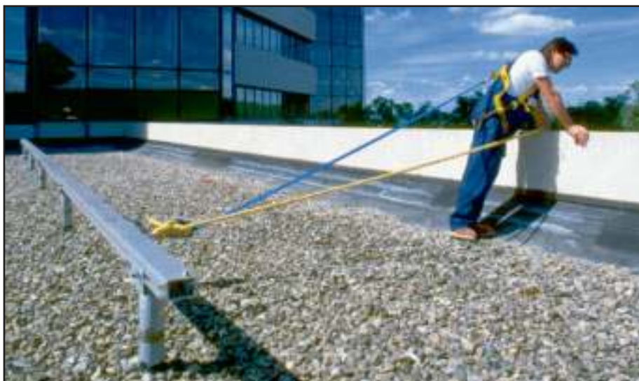
Roof mounted horizontal aluminum rail. Photo shows worker preparing to work over parapet. Both lines are secured to rolling trolleys. Parapet to support 1800 lbs (7.9 kN) vertical load.
