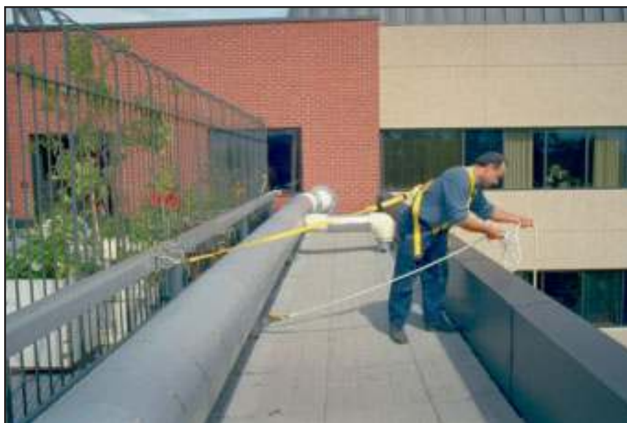
Pier mounted horizontal steel rail with rolling trolleys provides continuous horizontal movement for workers. Yellow lanyard restricts travel to inside of the low parapet which is less than 42" (1067 mm) guard rail height. Safety anchors at base of air duct are used to secure bosun's chair suspension line and separate lifeline.
