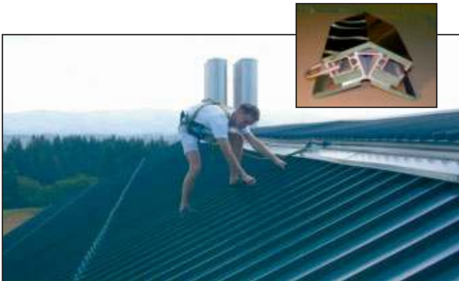
Photo shows a Pro-Bel ridge mounted type of trolley rail designed for the maintenance of a peaked roof. Worker's safety lifeline is secured to a stainless steel U-bar trolley located either side of the rail. The worker or several workers are able to traverse horizontally to any point on the roof, W.S.U. Physical Plant, Washington State University. Inset is product design photo of trolley rail.
