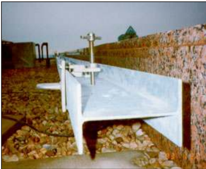
Pier mounted steel rail showing trolleys consisting of rollers, S.S. U-bar and T-type lock.
