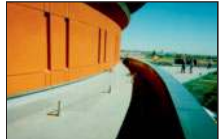
Lifeline application on narrow roof area with low parapet.
