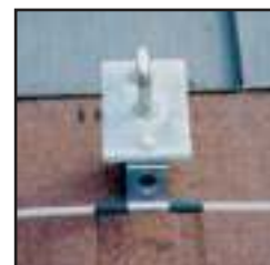
"Hands-Free" cable supports are often designed with a U-bar safety anchor for direct rigging of a bosun's chair.
