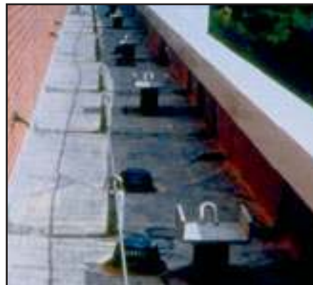
Photo shows Pro-Bel DL Horizontal Cable Lifeline system which employs double lanyard method of providing 100% tie-off. Parapet in this narrow roof area is less than 42" (1067 mm) safety guardrail height.
