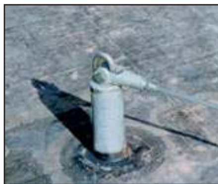
Photo shows terminal end of permanently installed DL Horizontal Cable Lifeline System. Swaged connection (shown) is at one end and a turnbuckle tensioner at opposite end.
