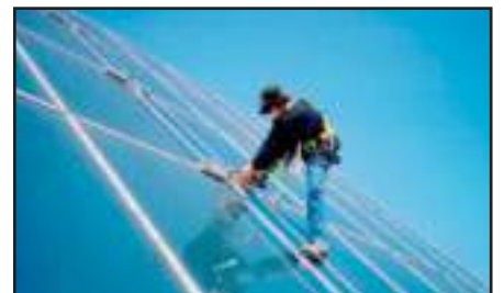
Worker changing to second lanyard while traversing DL Horizontal Lifeline up sloped atrium. Intelsat Global Service Corporation, Washington, D.C.
