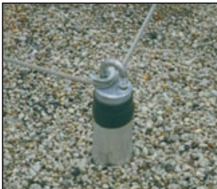
Corner anchors are used with a double lanyard system when changing direction. Anchors are typically placed at the same distance from the roof edge.
