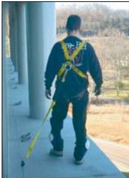
Worker above uses Pro-Bel "Hands-Free" Horizontal Lifeline Cable to safely access recessed windows as well as custom ledge-mounted Pro-Bel safety anchors (one for bosun's chair and one for lifeline) for "drops" as indicated at right, which shows four window cleaners working same facade.
