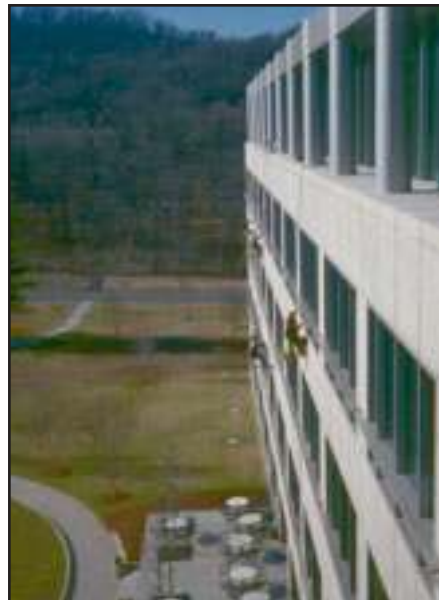
Worker above uses Pro-Bel "Hands-Free" Horizontal Lifeline Cable to safely access recessed windows as well as custom ledge-mounted Pro-Bel safety anchors (one for bosun's chair and one for lifeline) for "drops" as indicated at right, which shows four window cleaners working same facade.
