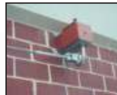
End swage connected to terminal U-bar anchor which is welded to structural steel penetrating a masonry wall.
