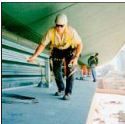
Workers traversing spandrel ledge under sloped roof canopy using DL Horizontal Cable Lifeline system (post mounted).
