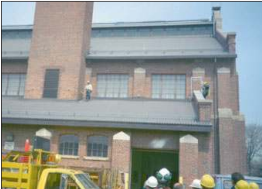
Pro-Bel "Hands-Free" Cable Lifeline system is used for window cleaning, roof inspection and similar maintenance. Vertical cable system is used with both access ladders at right to reach both roof levels safely.
