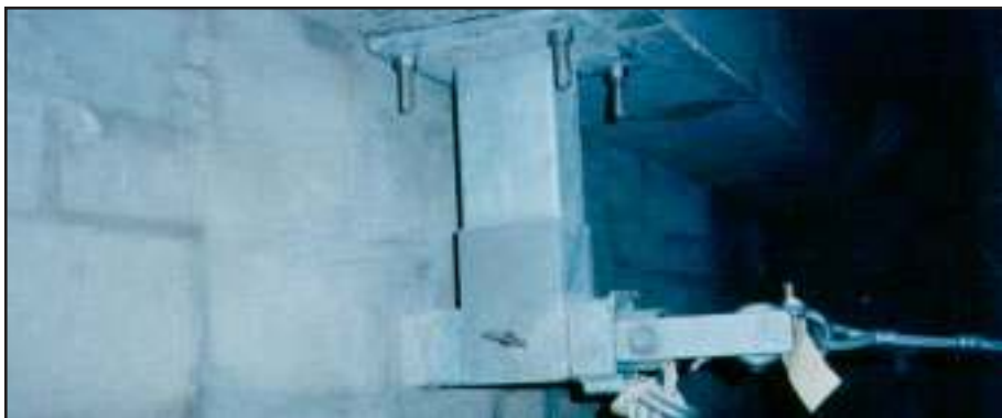
Horizontal rigging sleeve (in service position) is anchored to concrete roof beam and tied back to an interior wall mount safety anchor using steel cable. Worker's rope lifeline, tied to U-bar safety anchor, passes through sleeve to exterior.
