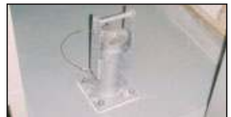
Pro-Bel roof-type rigging sleeve adapted for use in concrete floor.
