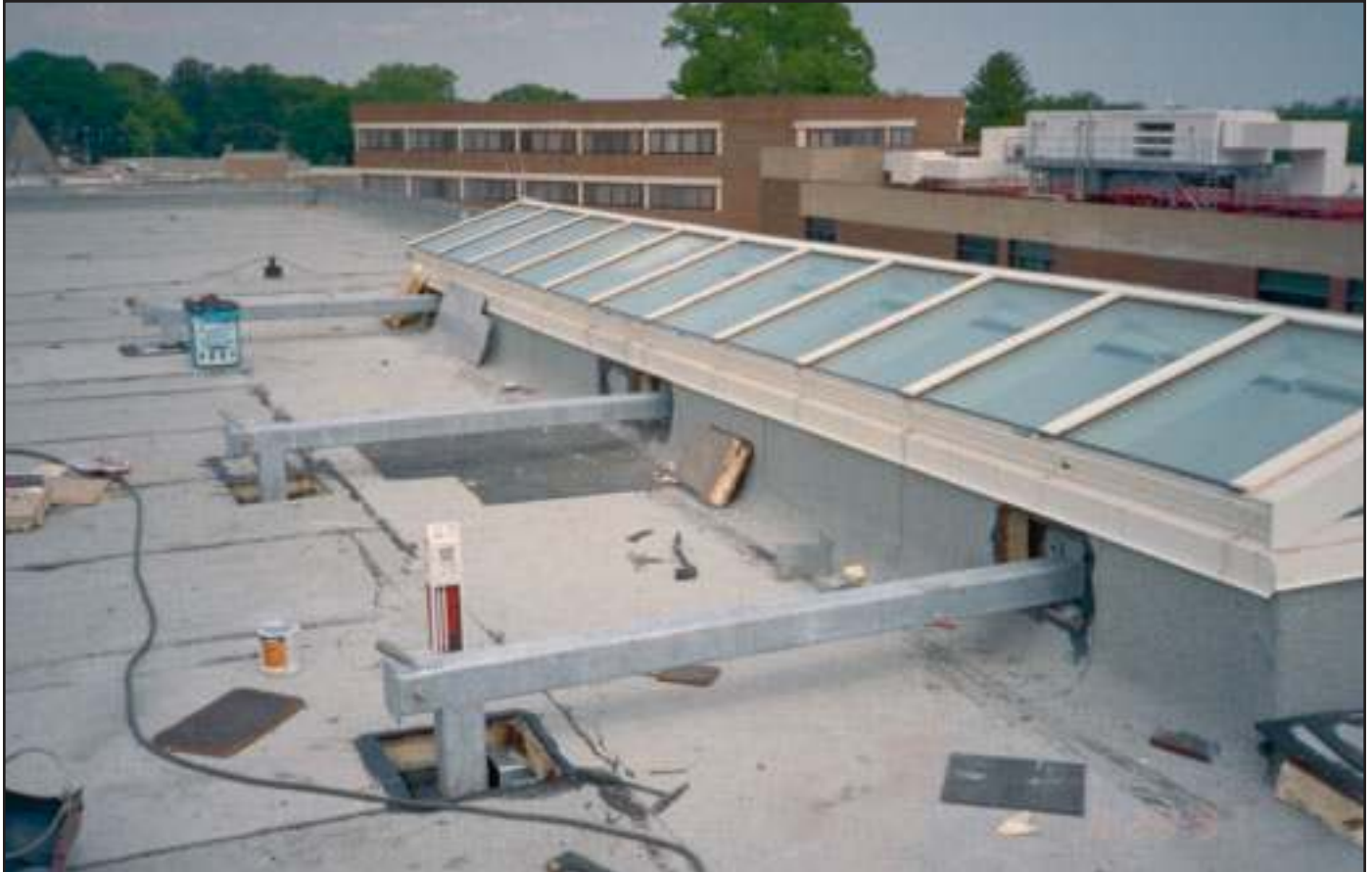
This retrofit application shows rigging sleeves being installed to service interior atrium windows using a platform. A long sleeve was required so that the pedestal at the rear of the sleeve could be welded to a structural roof beam. Lower right hand photo, in a different location, employs a shorter sleeve due to the location of the roof beam. In either case, the primary suspension lines are shackled to a straight bar at the rear of the sleeve and the worker's lifeline is secured to a U-bar at the rear of the sleeve and fished through the sleeve to the atrium floor below. University of Delaware College of Business and Economics, Newark, Delaware.
