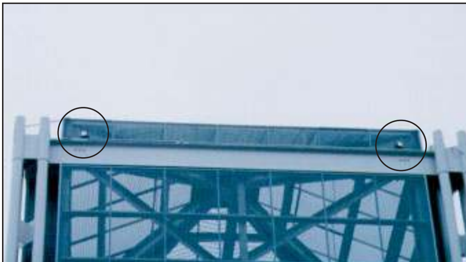
Rigging sleeves (circled) in this application were used solely to facilitate site painting of the structural steel in two tower structures. Pearson International Airport, Toronto.
