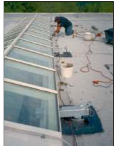
This retrofit application shows rigging sleeves being installed to service interior atrium windows using a platform. A long sleeve was required so that the pedestal at the rear of the sleeve could be welded to a structural roof beam. Lower right hand photo, in a different location, employs a shorter sleeve due to the location of the roof beam. In either case, the primary suspension lines are shackled to a straight bar at the rear of the sleeve and the worker's lifeline is secured to a U-bar at the rear of the sleeve and fished through the sleeve to the atrium floor below. University of Delaware College of Business and Economics, Newark, Delaware.
