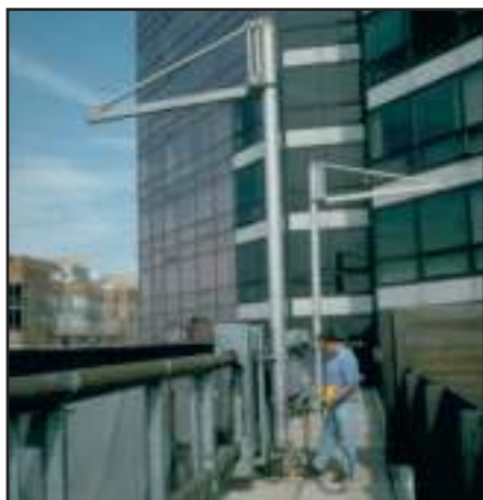
Motorized rolling davit system utilizing tubular wall mount tracks.
