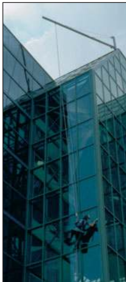
Working down face of building using Pro-Bel long span davit boom and bosun's chair. Bull Corporate Centre, Toronto, Ontario.
