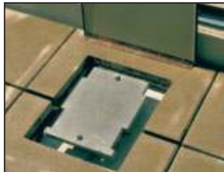
1. Concealed galvanized steel base is accessed by removing fitted metal cover plate.
