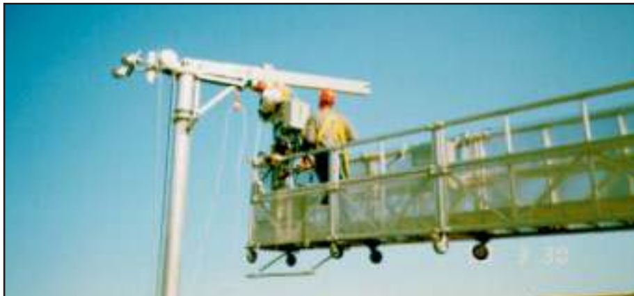
This photo shows Pro-Bel installers maintaining the manual chain driven trolley during the roof rigging process. U.C. Davis Medical Center, Sacramento, California.
