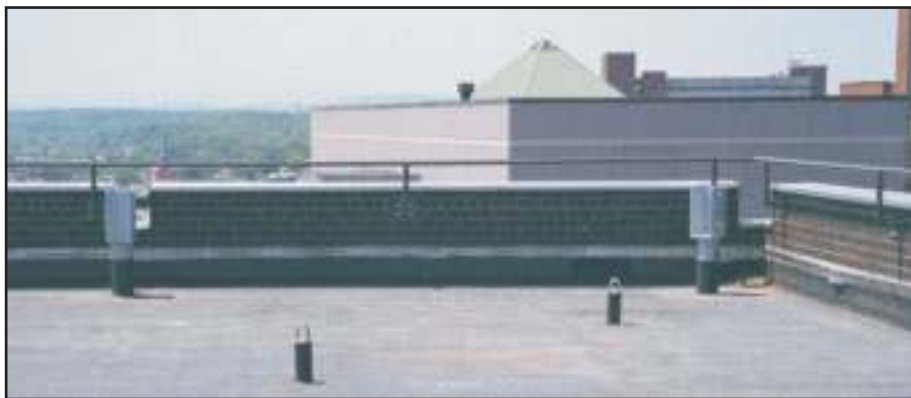
Davit bases (next to parapet) require separate and independent lifeline anchors (foreground).
