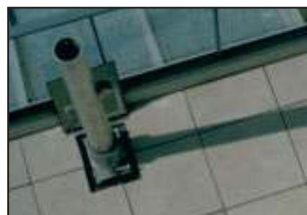
3. Aluminum mast is set into socket and twist locked into place.
