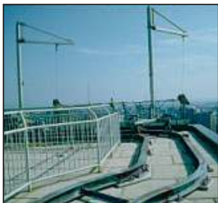
Motorized rolling davit system utilizing I-beam tracks.
