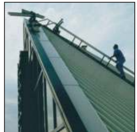
Ground rigged davit assemblies with permanent rotating heads and portable booms.
