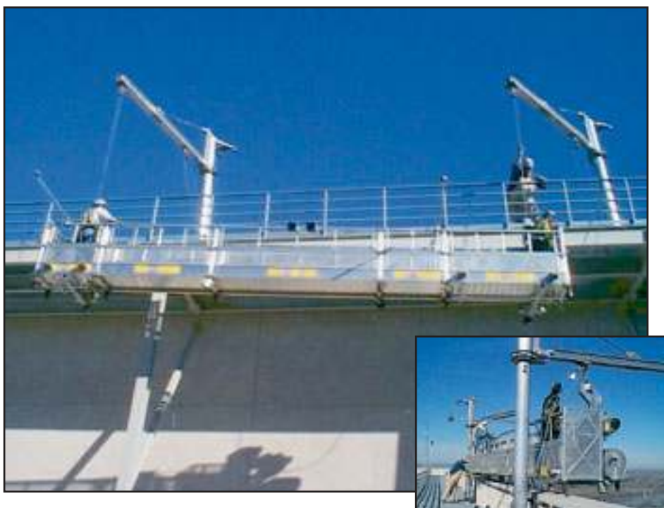
Pro-Bel long span roof rigged davit arms are used to hoist a platform from its storage location on a cooling tower roof and then swung across a wide metal catwalk and parapet over the side of the building. U.S. Courthouse & Federal Building, Sacramento, California.
