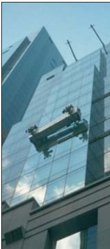
Long 14'-0" (4.3 m) span davit booms are employed to clear roof terraces, projections and lower levels. The Millennium building, New York, NY.
