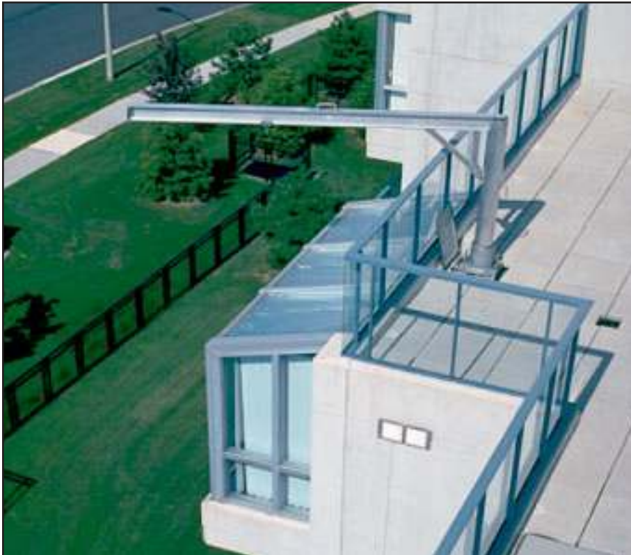
This long span aluminum davit boom was designed to circumvent a projecting sun porch.
