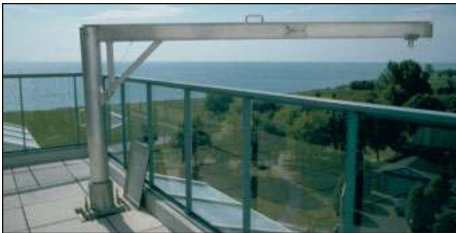
Recessed portable ground rigged davit. See assembly sequence at right.
