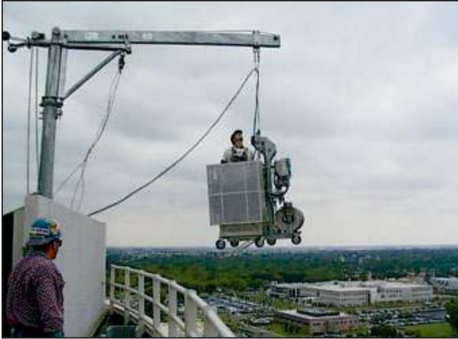
Pro-Bel permanent davit arm is used to clear high parapet rail and is suited to both single work cage and permanent powered platform. UC Davis Medical Center, Sacramento, California.
