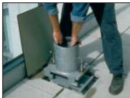
2. Galvanized mast socket is secured to base via lugs and spring-loaded locking devices.
