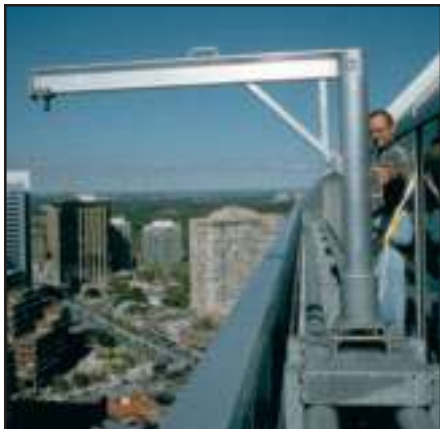
Rolling davits are designed for roofs with restricted access or long reach rigging options. Worker is shown manually positioning davit. Motorized models are also available. Worker's lanyard is clipped to U-bar safety anchor welded to rolling carriage. 25 Sheppard Ave., Toronto, Ontario.
