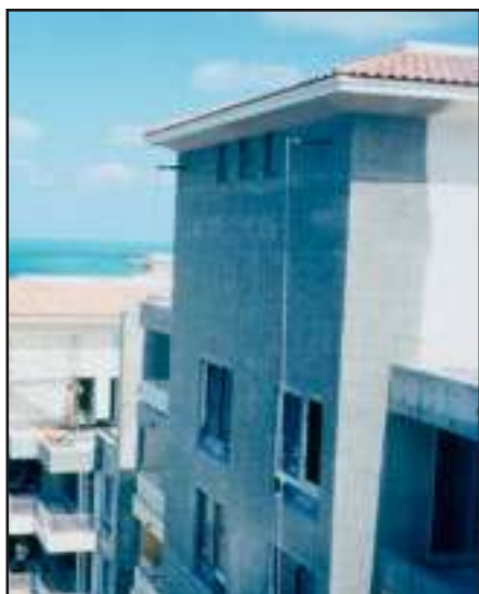
Photo shows wall sleeve application. When not in service, rigging sleeves retract to interior of building. Wall is stucco finished masonry. See close-up photo at right.
