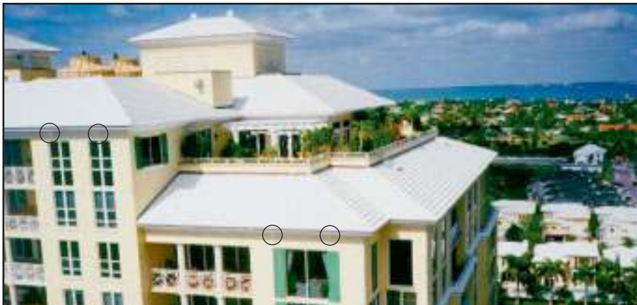
Curved rigging sleeves projecting from soffit (circled areas) are used to provide suspension points for platform and worker lifelines for window cleaning of non-balcony windows. Grand Bay Residences, Key Biscayne, Florida.
