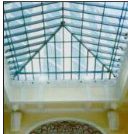
Perimeter skylight monorail system is used to service interior glass atrium and interior lighting system. Monorail corner-turning hubs are utilized to facilitate automatic turning at corners.
