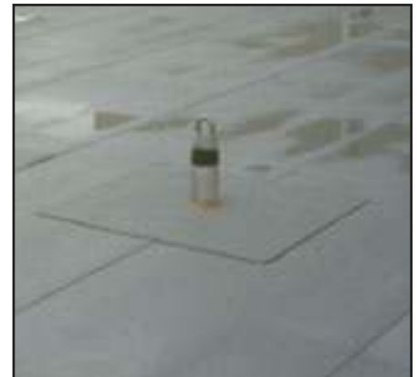
Single ply roof showing typical Pro-Bel roof anchor. Reliable flashing/sealing techniques are employed to satisfy virtually any roof membrane condition.
