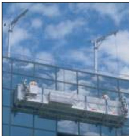
Pro-Bel modular powered platform system suspended from roof rigged davits.
