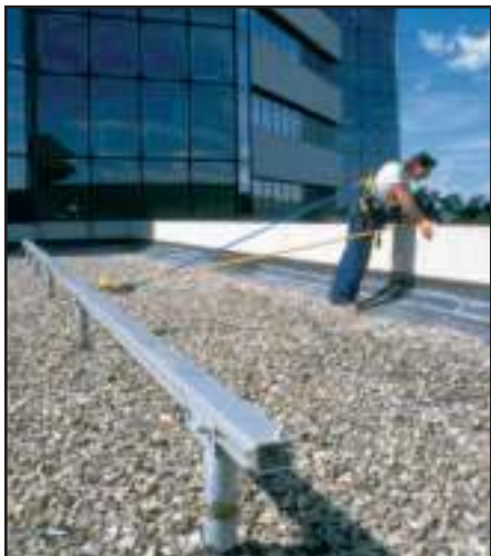
Monorail can also be roof mounted (as shown) or wall mounted to suit application.
