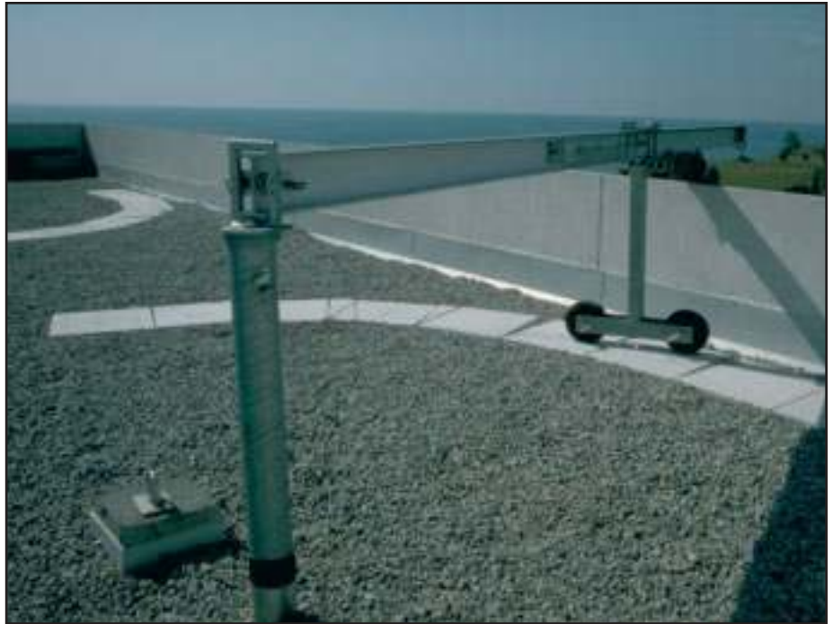
Pro-Bel portable swivel-type outrigger beam with dolly is designed to suit a specific roof area and can be relocated within the dedicated work zone. Portable systems must be pinned to permanently installed bases or anchors during maintenance operations.
