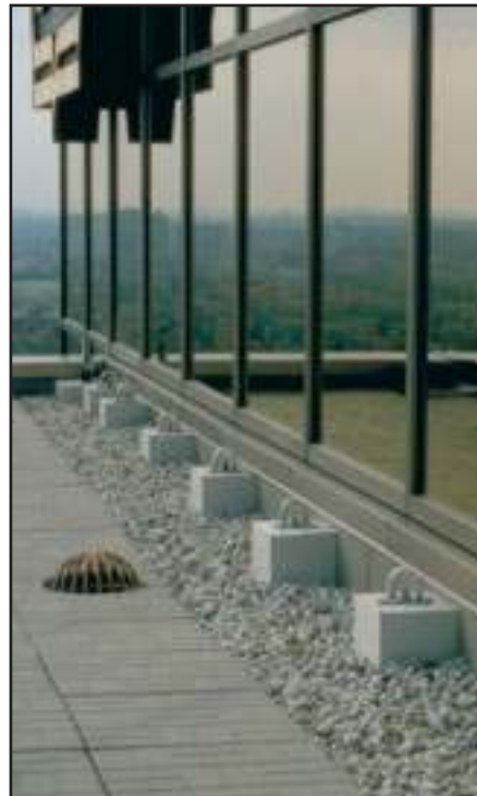
Planning of anchors should be incorporated during construction and designed to suit professional window cleaning and other building maintenance professions.
