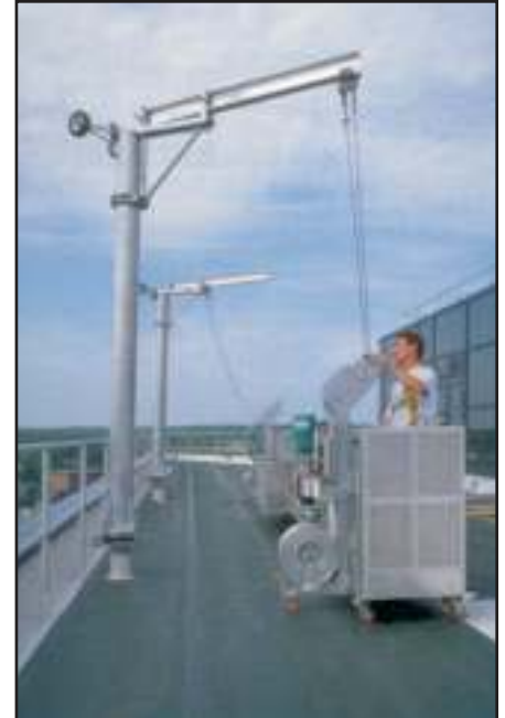
Pro-Bel roof rigged davits with modular powered platform system.
