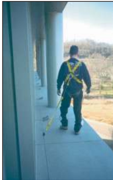
Worker above uses horizontal cable to safely access recessed windows as well as custom, ledge mounted Pro-Bel safety anchors for access to next "drop" using a bosun's chair. See photo below.
