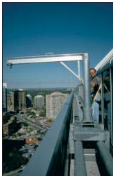
Pro-Bel rolling davit is designed for areas with restricted inboard space, access or rigging options.
