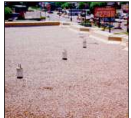
Due to stringent government standards, anchor placement requirements i.e. in line with the point of suspension and free fall distance, anchors must often be placed on the roof.
